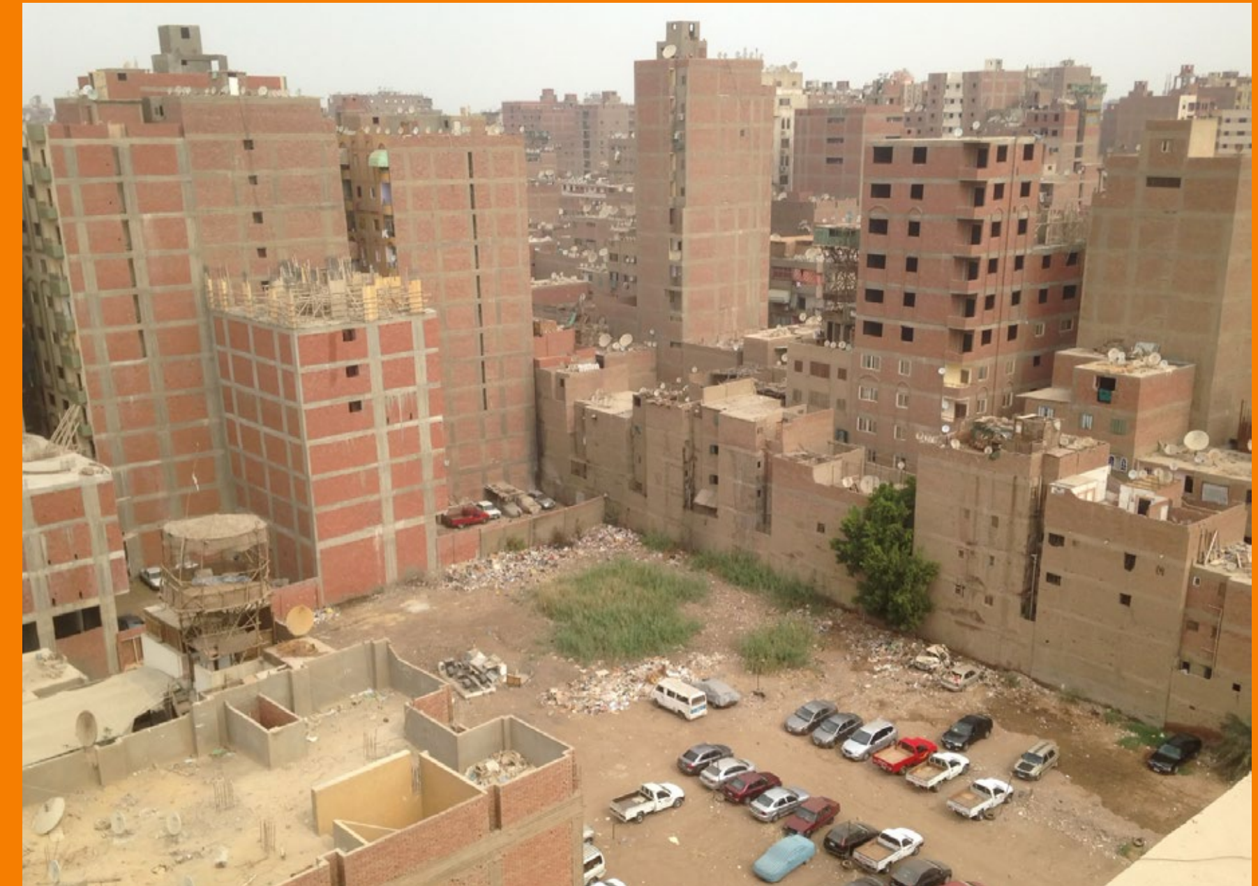
A typical informal housing block in the neighbourhood of Ard al-Liwa, Giza
